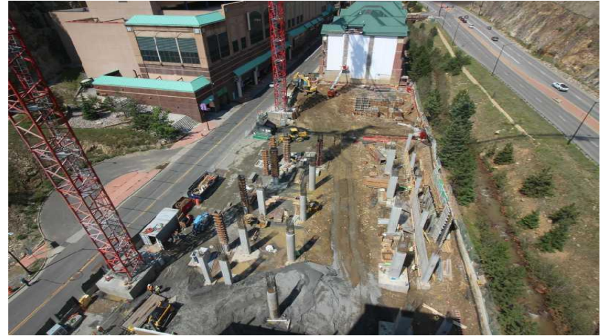
Hotel Tower/Casino Expansion: Current Progress
